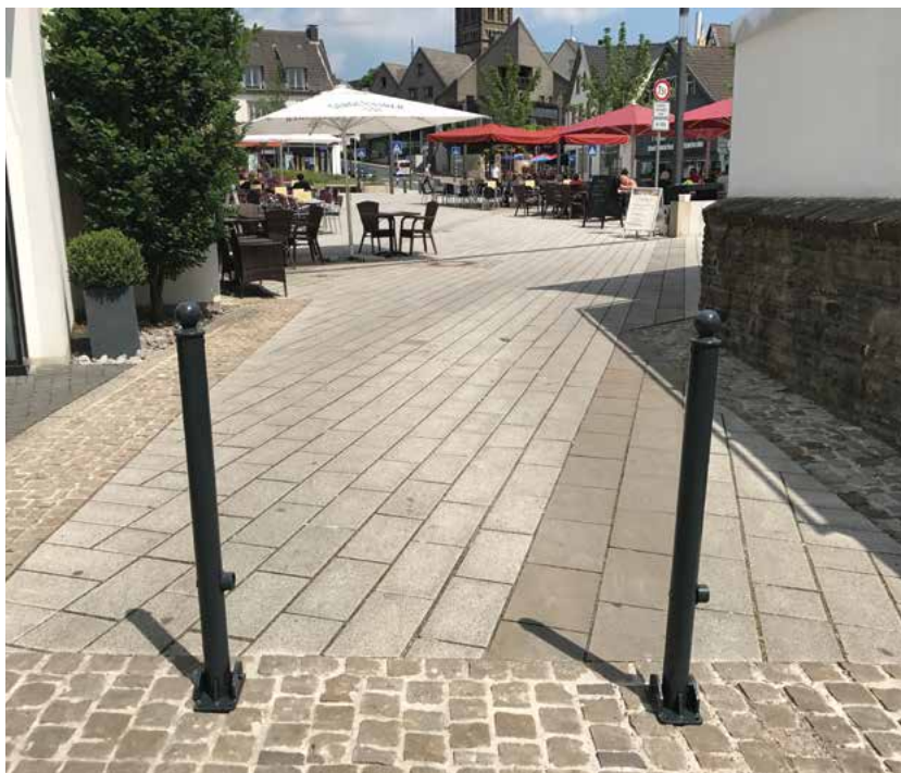
Ornamental bollard of steel tube Ø 60 mm approx. 950 mm above ground, hot-dip galvanized and coated
